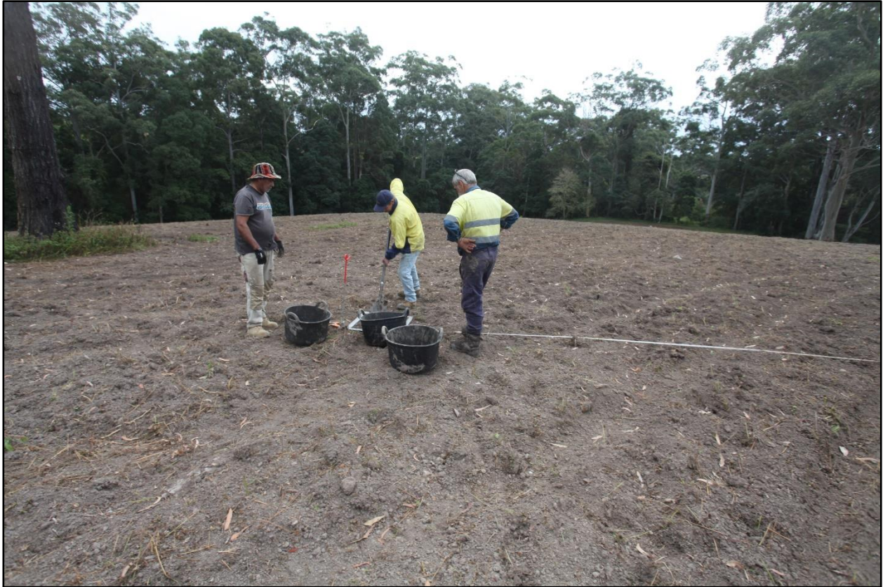
Figure 22: Test Pit 13- Excavation
